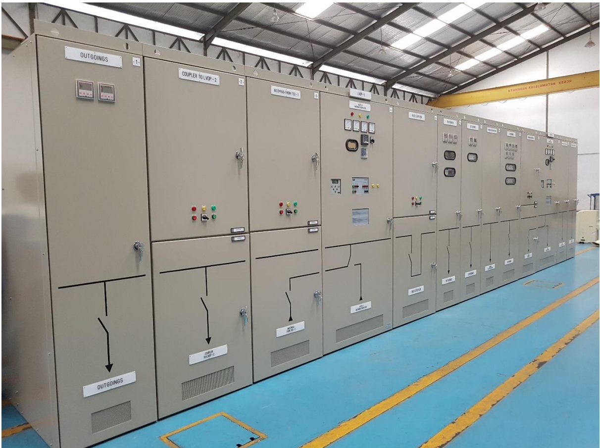
GE SENPlus 400V Motor Control Center Fully Drawout Type
