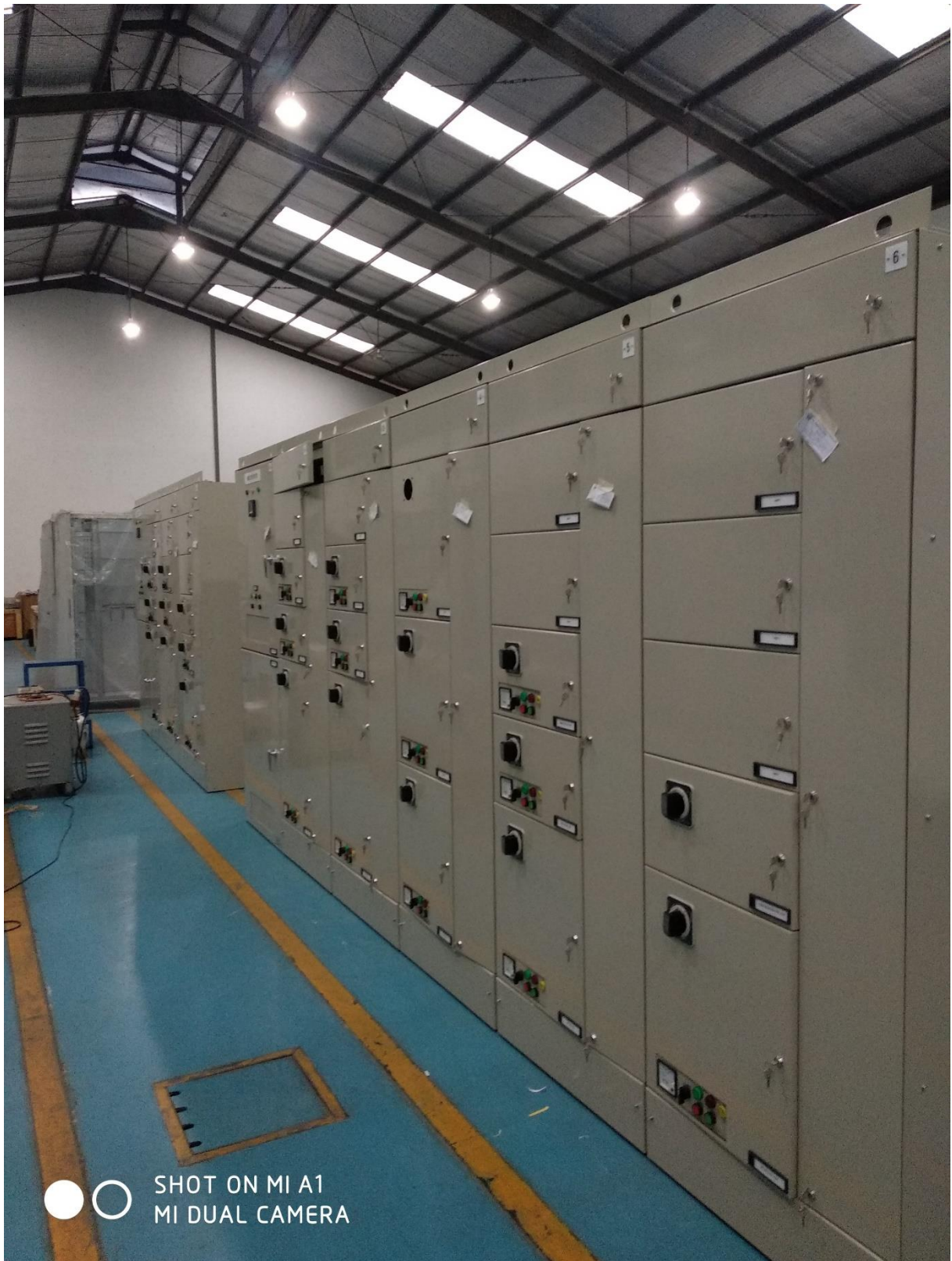
400V Motor Control Center Modular Fixed type
