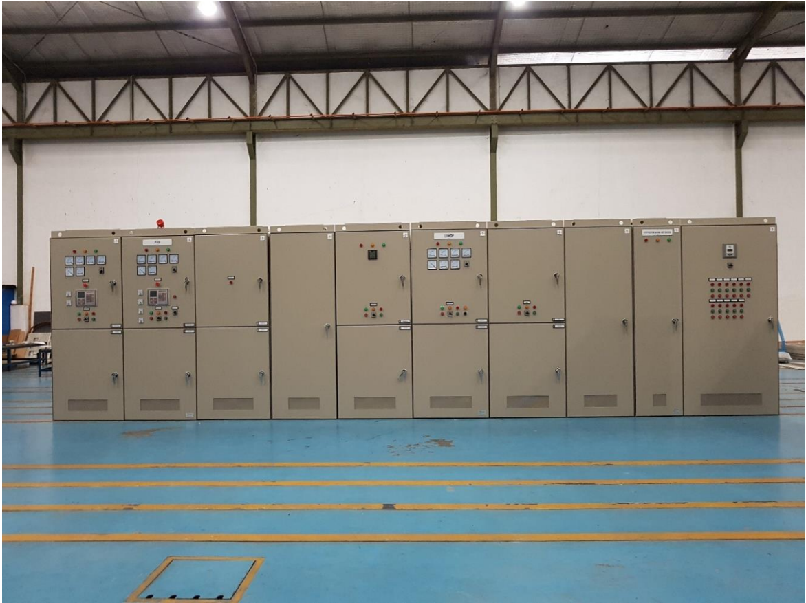
400V Switchgears , Auto Synchronizing Generator, Auto Transfer Switch (ATS) and Capacitor Bank
