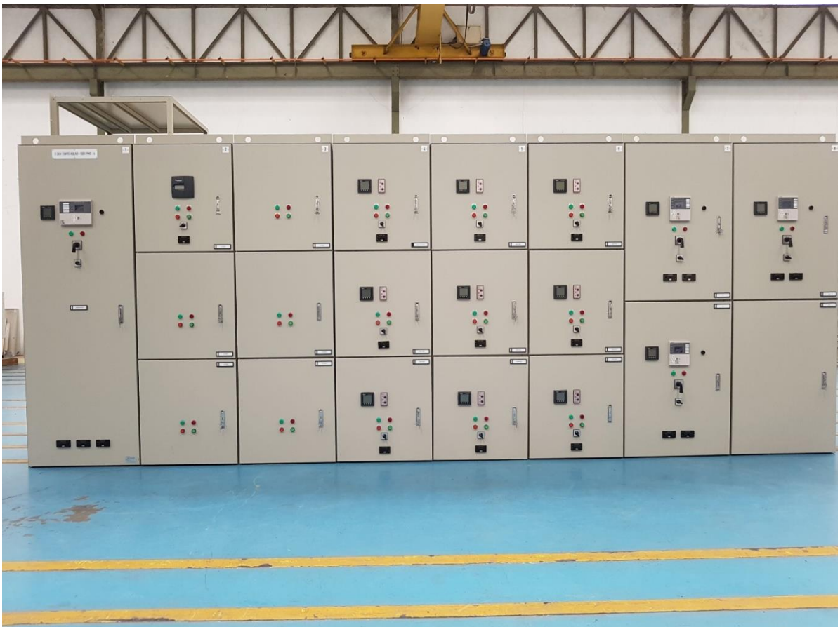
400V Switchgears , Auto Synchronizing Generator, Auto Transfer Switch (ATS) and Capacitor Bank
