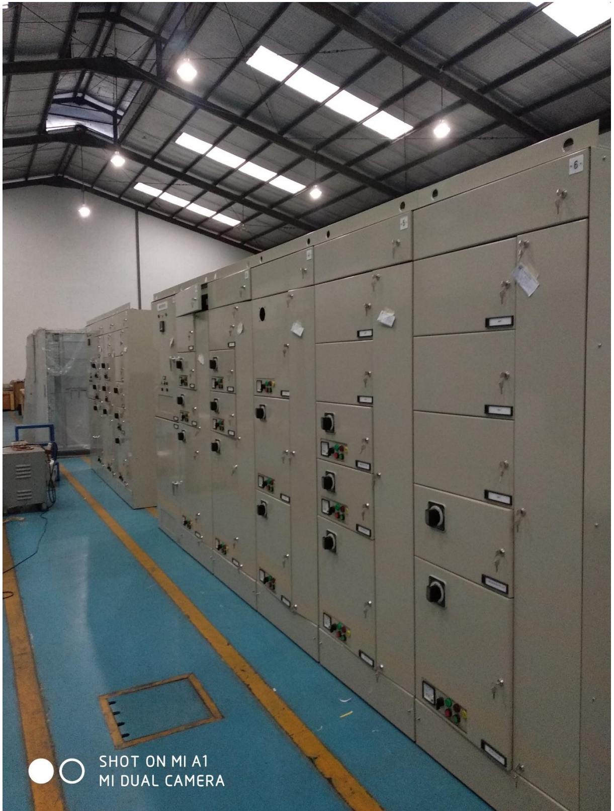
400V Motor Control Center Modular Fixed type
